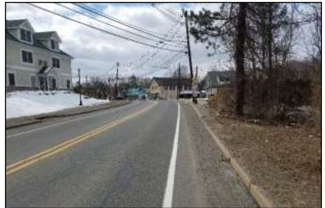
CR 620/98 Main St. : View of Project Site Looking West
